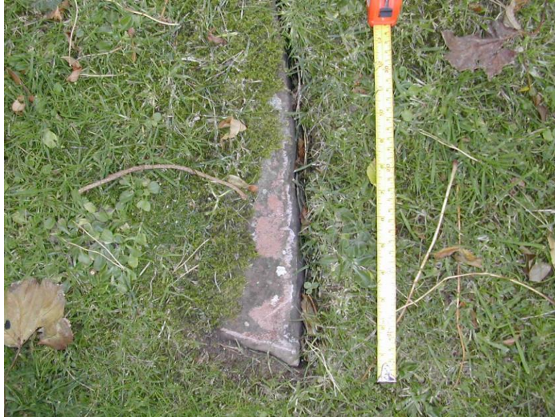
22. Recumbent slab damaged by strimming
