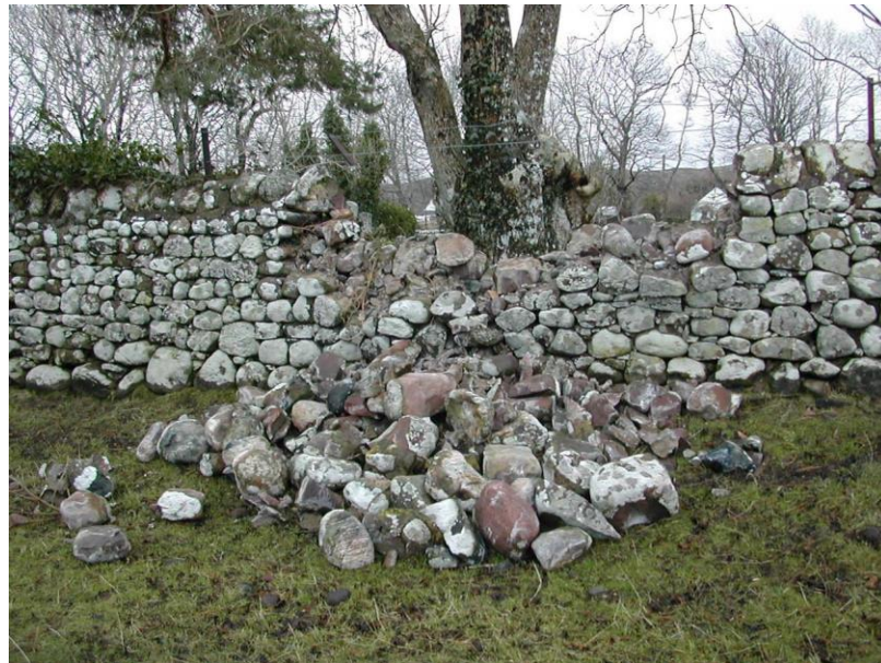
21. Tumbled wall, loosened by movement of tree roots during storm.
